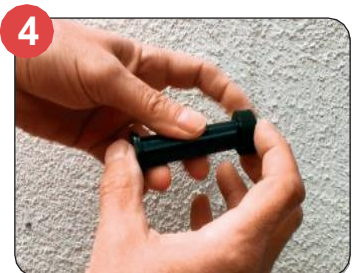
4 Place the neoprene washer onto tube and insert tube into wall.
