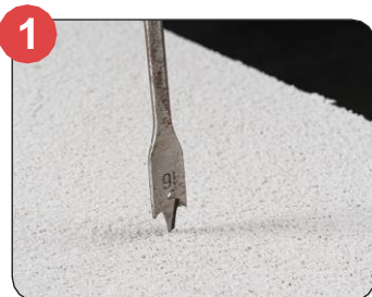
1 Drill a 16 -18mm hole through the render and insulation until the original substrate is reached.
