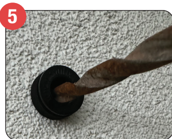
5 Drill the correct size hole and depth for the throughbolt through the tube, and clear debris from hole.
