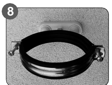
8 Secure the pipe clamp.
