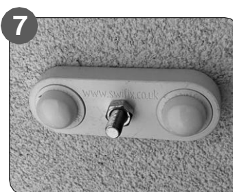
7 Insert plug, fixing and screw cap.
