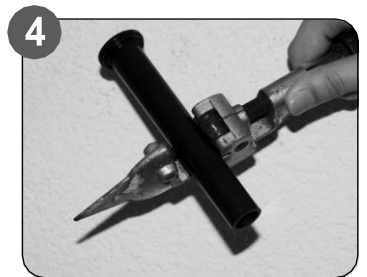
4 Cut tube to length using pipe cutter ensuring an allowance has been made for the dept of the plate.
