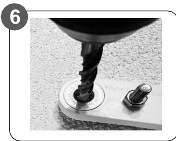
6 Drill through tube into substrate to the appropriate depth for fixing (site specific).
