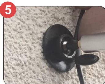
5 Insert screw utilising the screw cap fix item required (shown - p-clip attaching cable).
