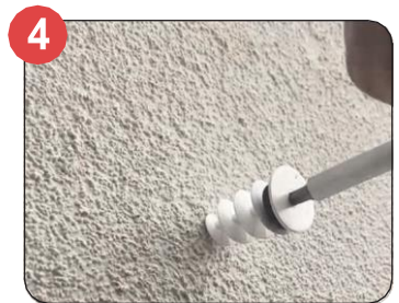
4 Carefully Screw into render using a T30 torx head screw driver. Note: Using mechanical means may burr the fitting.
