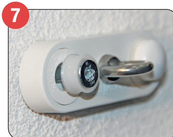
7 Insert plug, fixing and screw cap.
