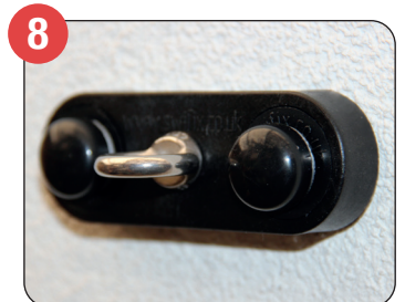
8 Secured and water tight.
