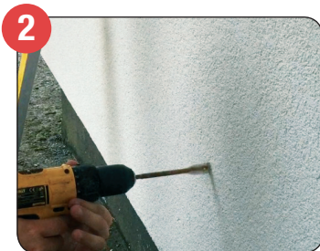
2 Drill a 16mm hole through the render and insulation until the original substrate is reached.
