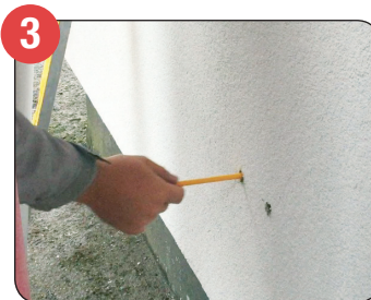
3 Insert tube, or measure depth of hole from finished render back to the original substrate, making an allowance of 4mm to allow the neoprene washer to compress and provide a seal when installed.
