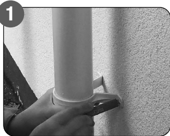
1 Mark the render to identify position of item to be secured.
