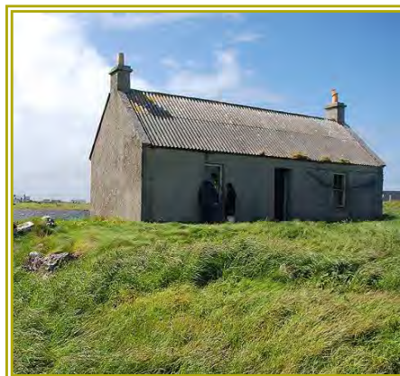
Stone cottage on Uist trial. Source: Locate Architects
