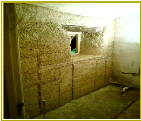
Hemp lime render on the slate cottage. Source: Centre for Alternative Technology
