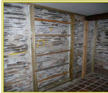
Wooden battens for internal wall insulation. Source: Centre for Alternative Technology
