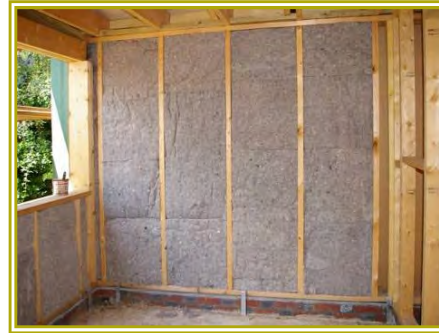
Hemp internal wall insulation. Source: Ecological Buildings Systems.
