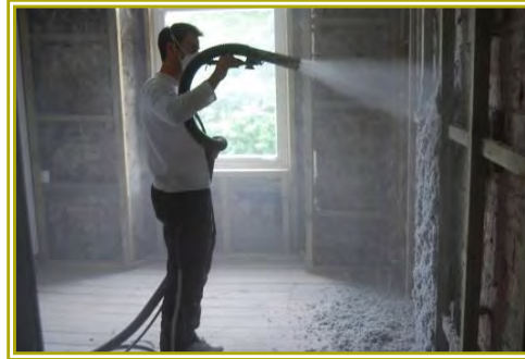
Cellulose fibre blown onto wall. Source: Historic Scotland presentation
