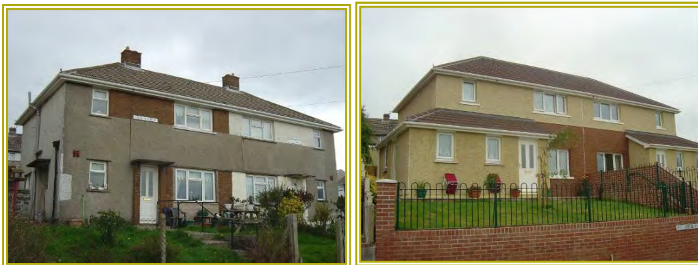
Before and after photos of a property with EWI. Source: Wetherby Building Systems Ltd
