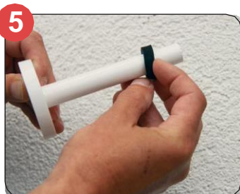
5 Place the neoprene washer onto tube and insert tube into wall.
