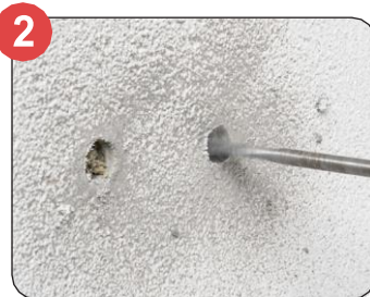
2 Drill a 16 -18mm hole through the render and insulation until the original substrate is reached.
