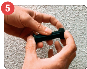
5 Place the neoprene washer onto tube and insert tube into wall.
