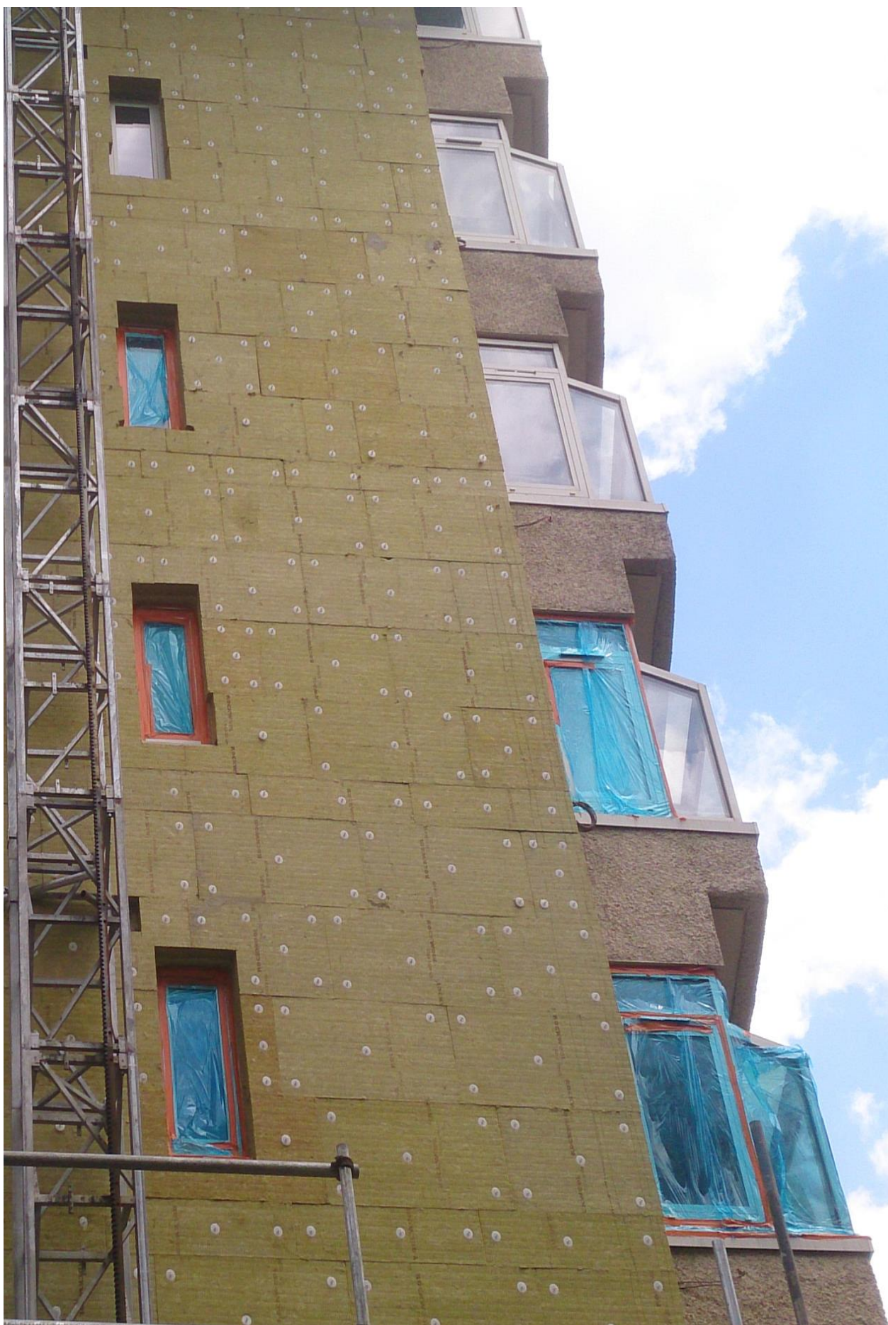
External insulation in progress to high-rise block
