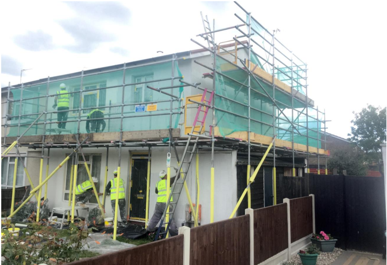
External SWI installation
