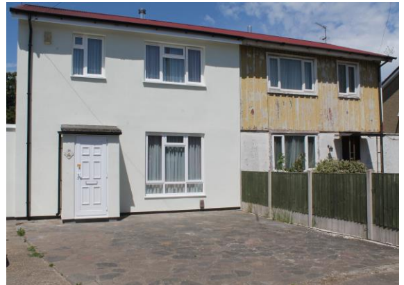
A BISF type system-built home from the 40s externally insulated alongside its neighbour
