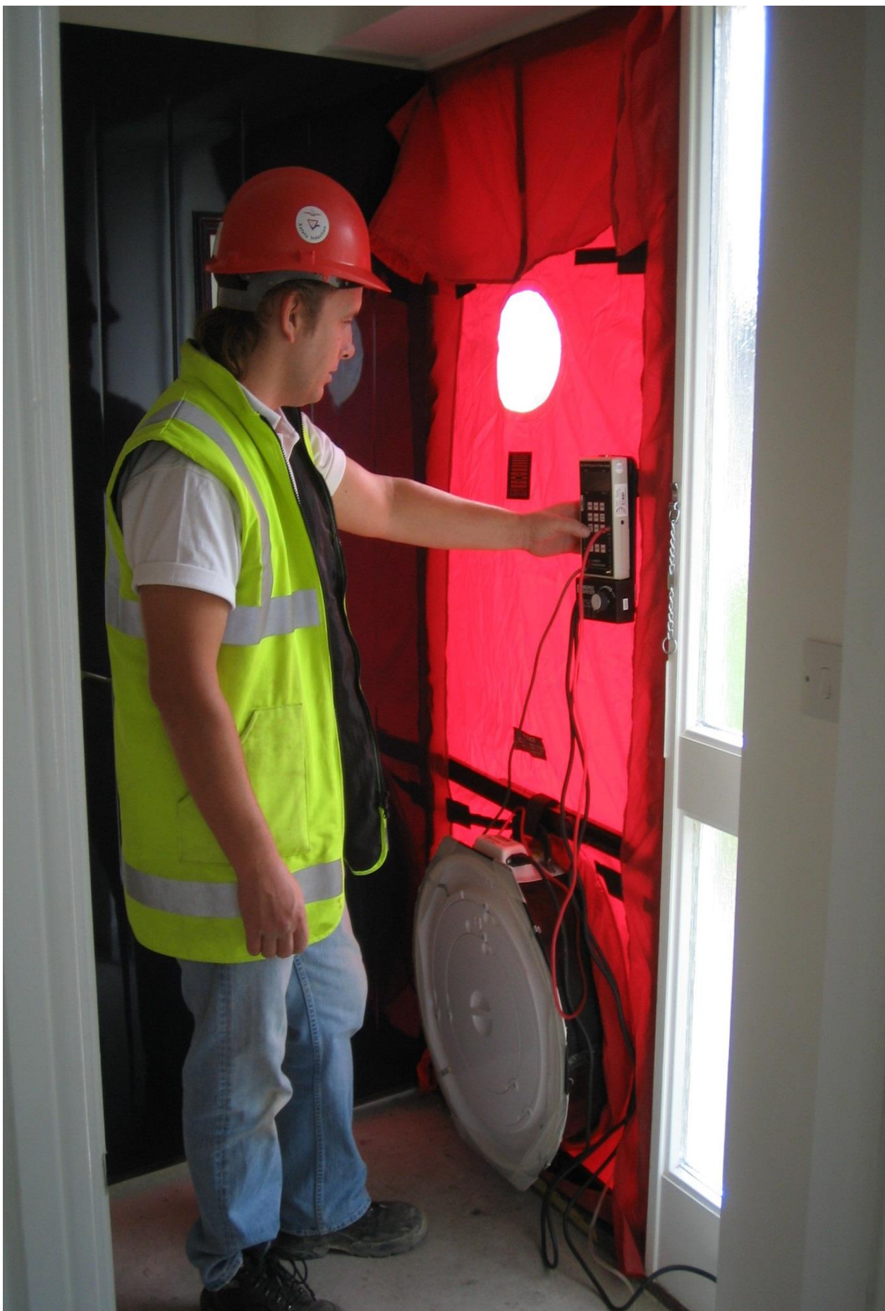
Air tightness testing
