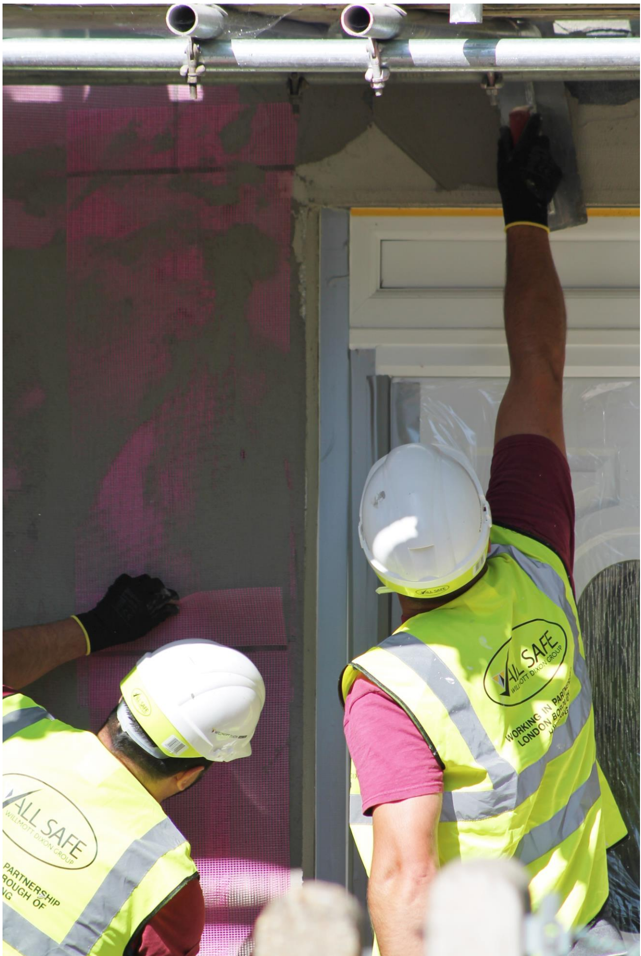
Applying wet trades
