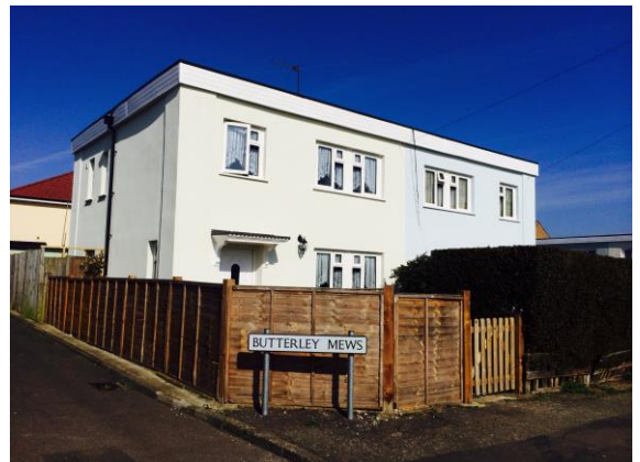
An Orlit type system-built home after external wall and roof insulation
