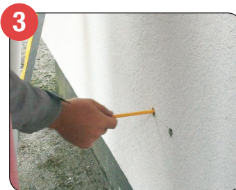
3 Insert tube, or measure depth of hole from finished render back to the original substrate, making an allowance of 4mm to allow the neoprene washer to compress and provide a seal when installed.
